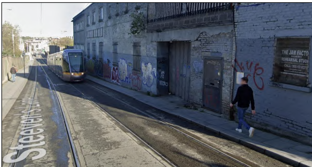
Figure 6. Narrow Section of Steeven's Lane Eastern Footpath
