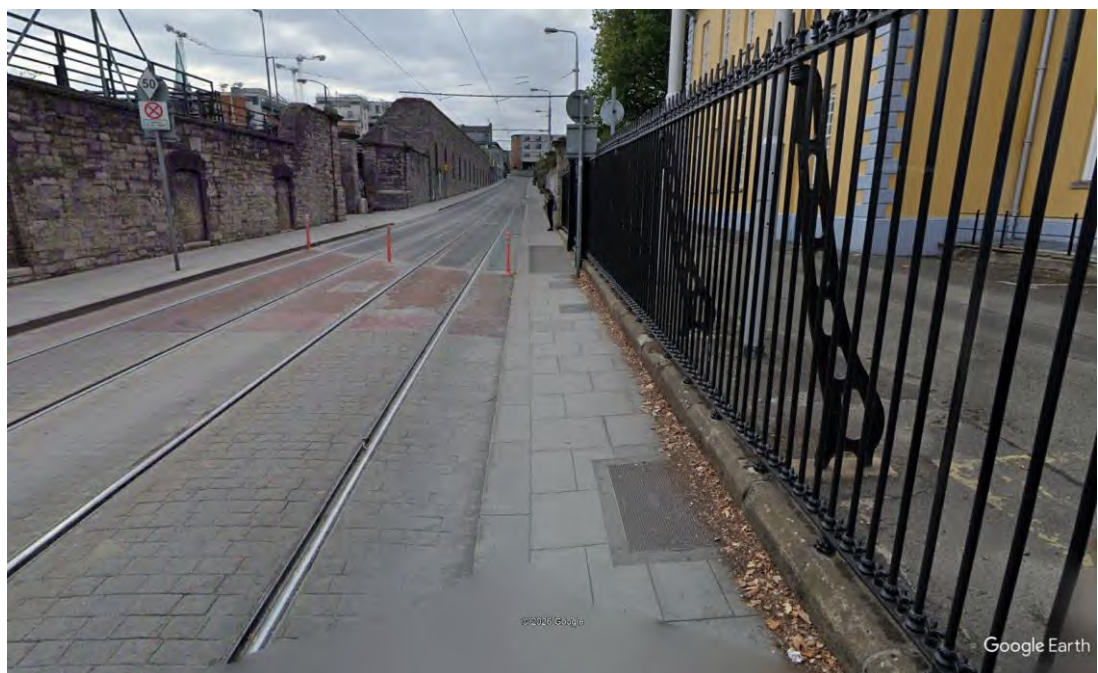
Figure 7. Narrow Section of Steeven's Lane Western Footpath
